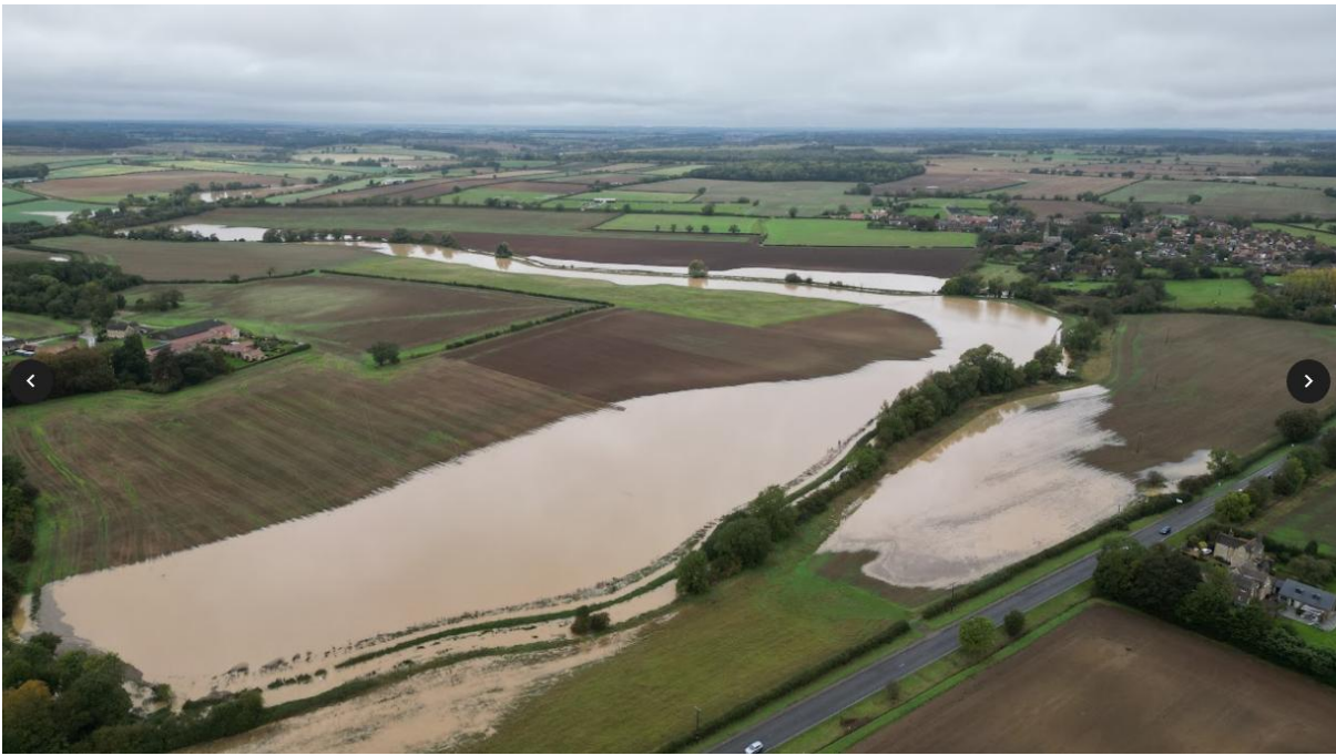
Showing river bank breached west of A6121 with Carlby village (top right)
